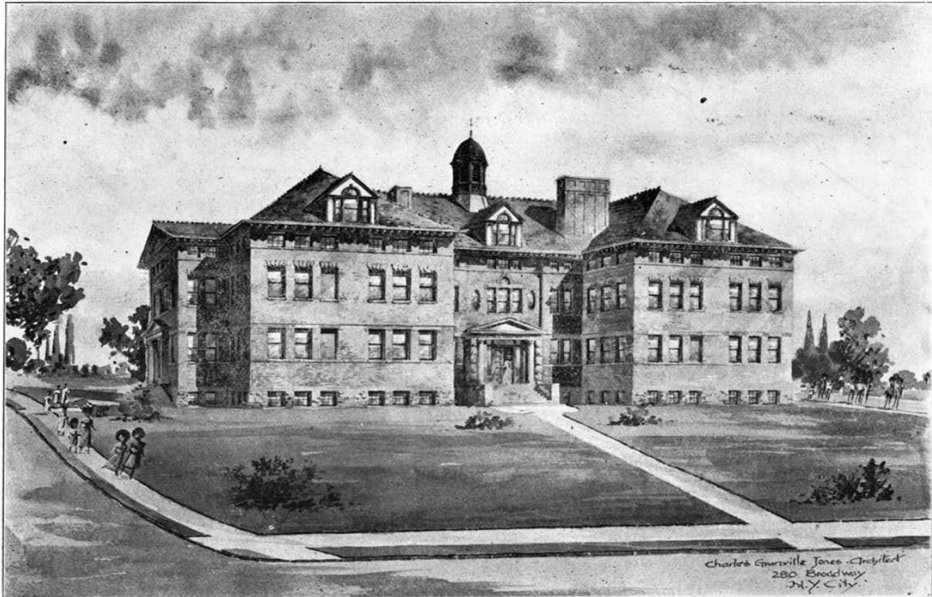
PARK SCHOOL, WITH ADDITION.
